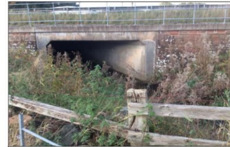
Photo Location 3: Culvert facing downstream
